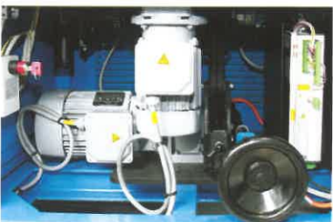
Main drive refurbishment.
